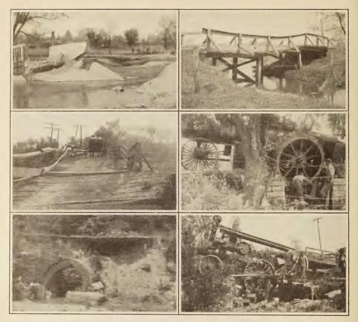
TOP LEFT—BRIDGE BUILT ON UNASSISTED LOCAL DESIGN. RIGHT—EVEN THIS COULD BE IMPROVED BY PROPER MAINTE-NANCE. CENTER, LEFT—UNSAFE BRIDGE WITH NO WARNING SIGN. RIGHT—HOW MUCH HAS THIS ACCIDENT COST THE OWNER OF THE TRACTOR? BOTTOM, LEFT—NO WARNING SIGN ON THIS DANGEROUS BRIDGE. RIGHT—PRIMITIVE FORM OF CONSTRUCTION CAUSES TROUBLE.
